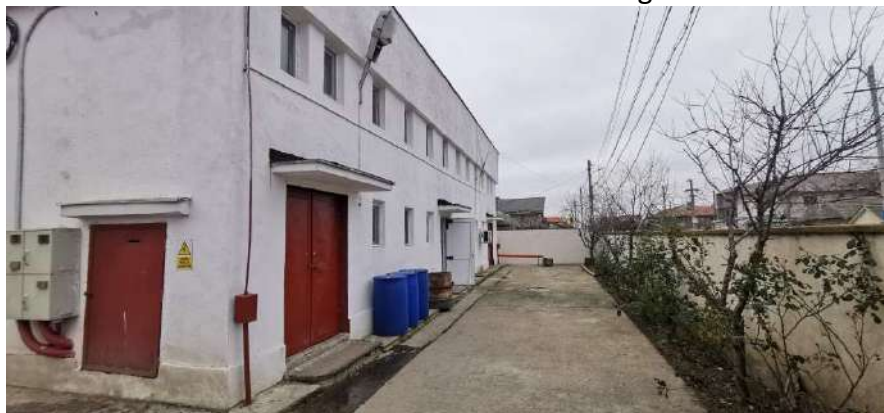
Fig. 5 The garage building section where SFD staff will be relocated
