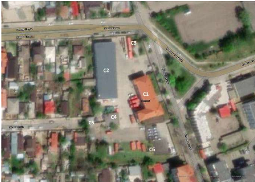
Fig 3 IESI and SFD's buildings satellite view
