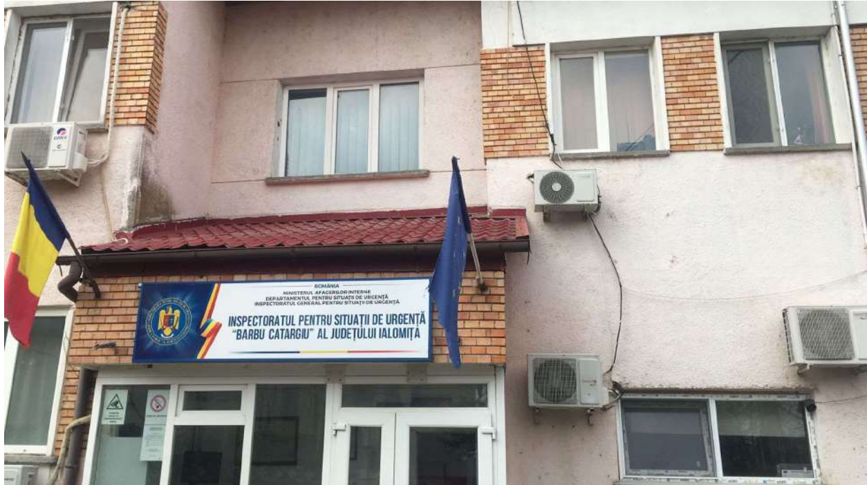
Fig 7 Existing IESI and SFD's C1 administrative building C1
